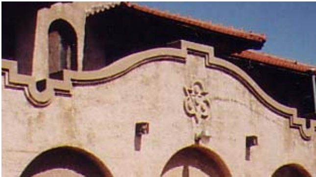
Mission-Revival style details used by the Santa Fe Railway included stucco, red tile roofs, rarched openings, emates and quatrefoils, like those found on this facade of the Gran Quivira Harvey House in Clovis.
