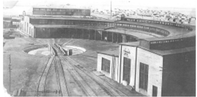
Clovis Roundhouse, circa 1926, demolished
